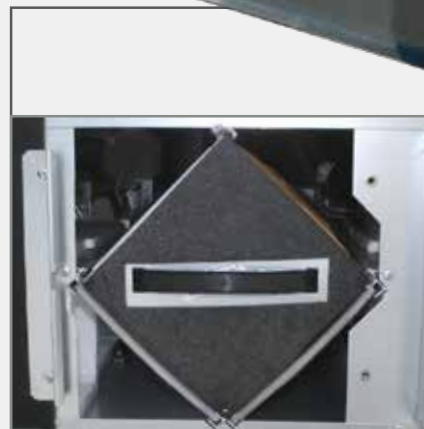
FILLING MATERIAL INSPECTION HATCH
